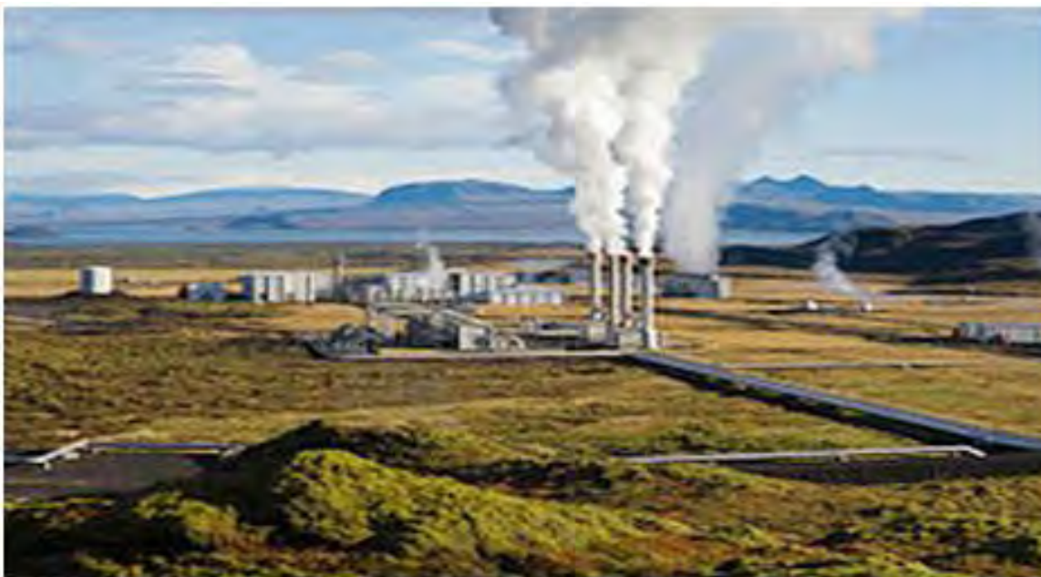
Steam rising from the Nesjavellir Geothermal Power Station in Iceland
